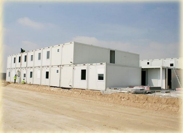
Container office in Brazil
